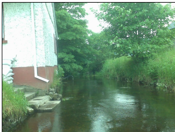
Photo 4: Existing Building adjacent to the Turnalaydan Stream at Lackagh Bridge
