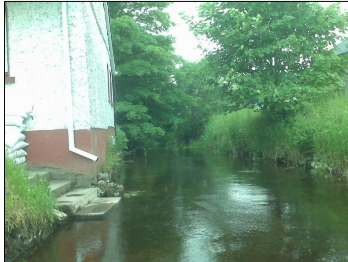
Photo: Existing House located adjacent to Turnalaydan Stream. Note the sandbags on the steps.
