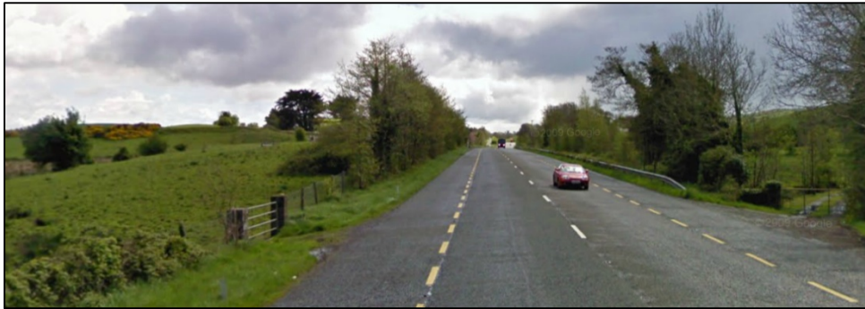
Photo 10: Location of the existing N4- Tributary of the Drumderry Stream Crossing
